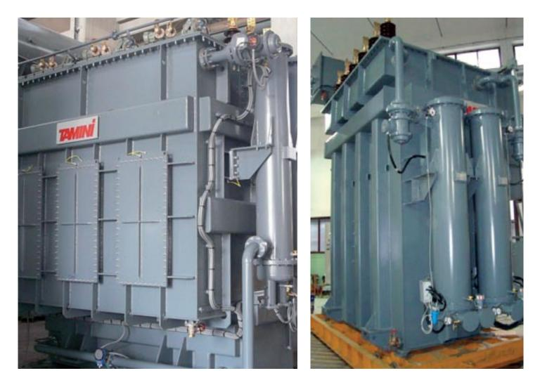
Tamini has designed and successfully supplied many different types of transformer - reactor solution. Among them the "Booster-type" one, in which the reactor is built-in, is the solution that optimizes the voltage/current values in the transformer regulation circuit.
